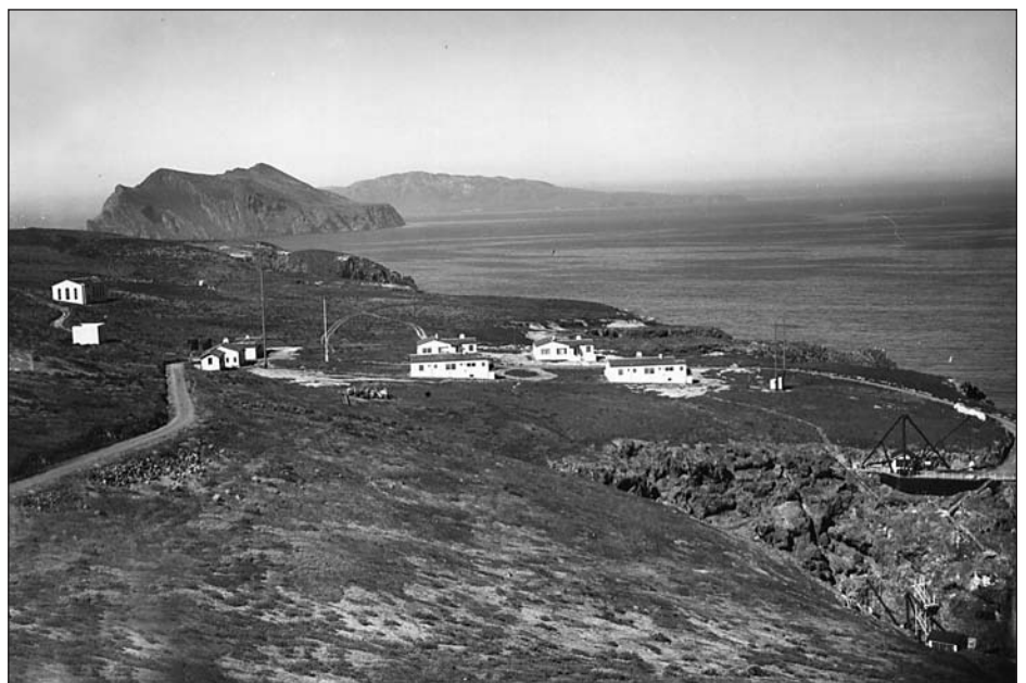
Anacapa Light Station. Looking west with Middle and West Anacapa Islands in the background. From left – power house, work shops, four dwellings and at extreme right the top area of the landing.
