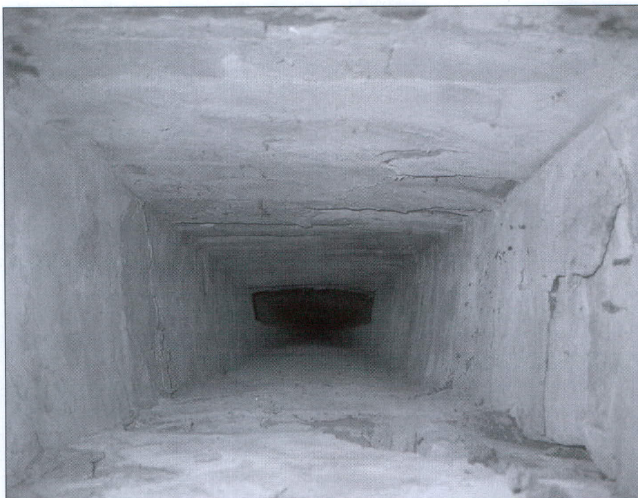
Two views of the weight shafts built into the walls of many lighthouses. Above, looking down the shaft, and below, looking up the shaft in another tower. Photos by the author.
