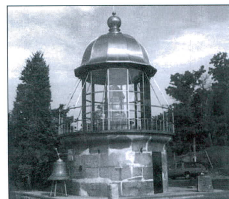
Below – Replica of Minots lantern room with what remains of the original lens. Photo courtesy of the author.
