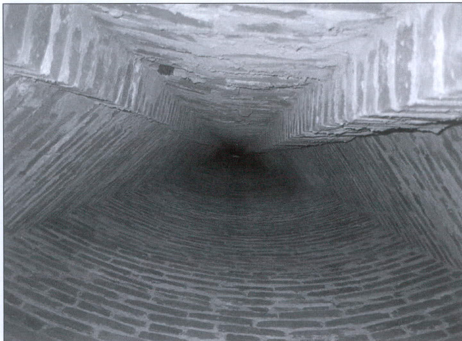
Two views of the weight shafts built into the walls of many lighthouses. Above, looking down the shaft, and below, looking up the shaft in another tower. Photos by the author.
