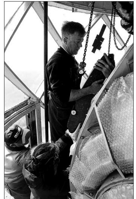
Volunteers dismantling the Fresnel lens for restoration in 1998. Photo courtesy of David Russell.
