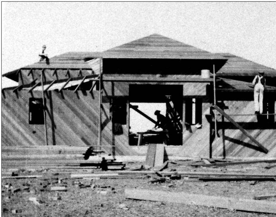
Construction of the station barn in 1909. Photo courtesy of the U. S. Coast Guard.
