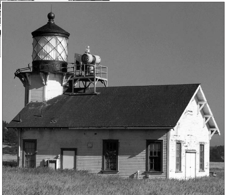
Below – The lighthouse (fog signal) building prior to restoration. Note the fog signals have been removed and the DCB-224 aero beacon on the roof. Photo courtesy of PCLK.
