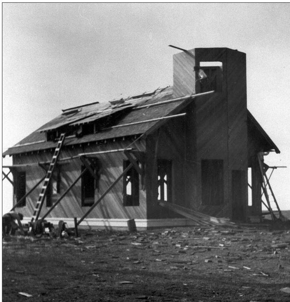
Above – Point Cabrillo Lighthouse under construction in 1909.
