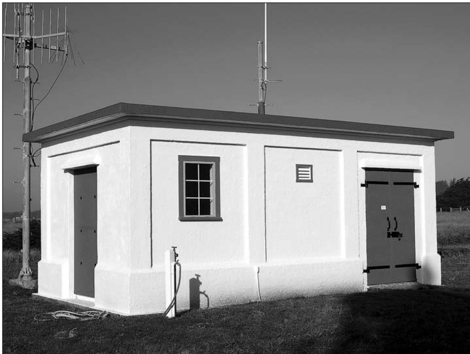
The oil house originally stored the kerosene oil for the lamps. It now contains the USCG VHF Repeater and Loran Monitoring Equipment. Note the antenna at left and on the roof. Photo courtesy of Bruce Rogerson.
