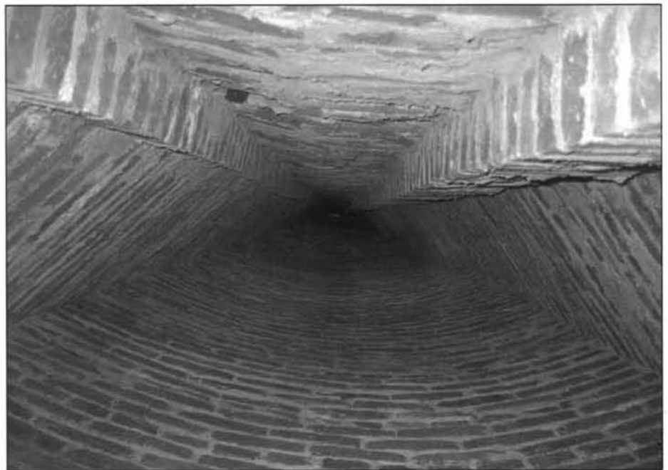
Two views of the weight shafts built into the walls of many lighthouses. Above, looking down the shaft, and below, looking up the shaft in another tower. Photos by the author.
