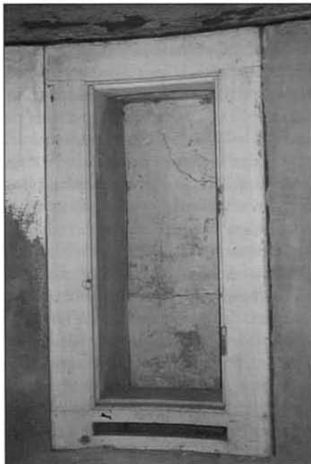
Door at the top of the weight shaft. Note the slot at bottom for the (missing) shelf. Photo by the author.
